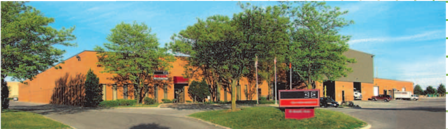
Our 145,000 sq. ft. design, manufacturing, and customer service facility in Concord, north of Toronto, Ontario
